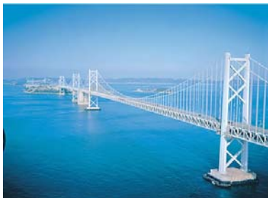
Seto Ohashi Bridge
